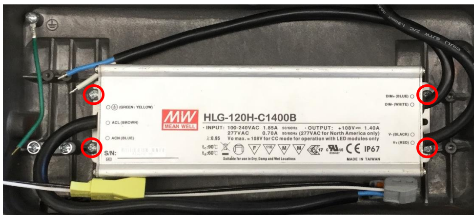
Figure 1: Remove (4) Screws Securing Driver
